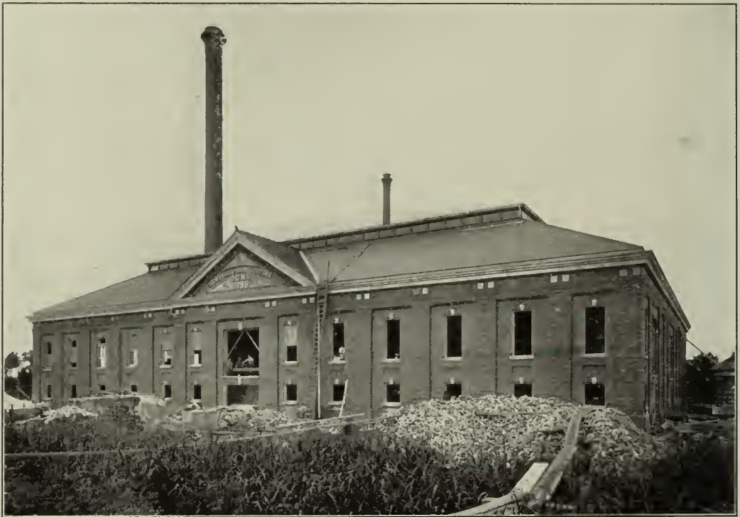
FRONT VIEW OF CENTRAL POWER HOUSE, IN COURSE OF ERECTION.
